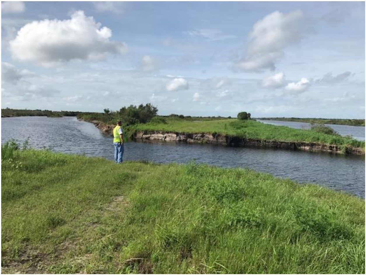
South end of triangle just south of S-65A lock structure on eastern side of Kissimmee River.
